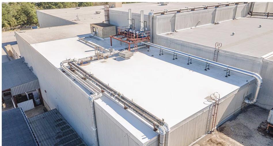
Trane Technologies manufacturing facility, Tyler, TX. This EverGuard Extreme® TPO 60-mil roofing system is approved under FM 4470 - Very Severe Hail (Class 1-VSH).
