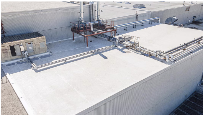
Trane Technologies manufacturing facility, Tyler, TX. EverGuard Extreme® TPO 60-mil roofing system.
