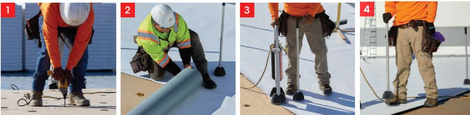
1 Attach insulation or cover boards to deck using Drill-Tec™ RhinoBond® Plates and Fasteners.
